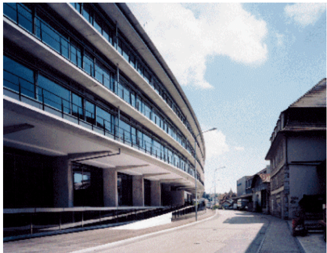
Figure 2.16: S-E facade of the OCH02 building
