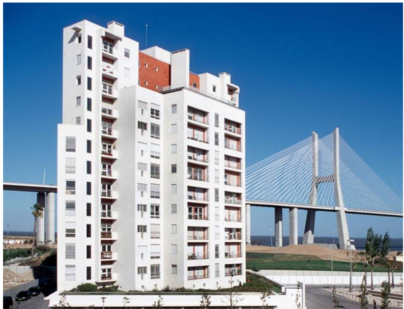
Figure 2.10: APT06 building on the Expo98 site
