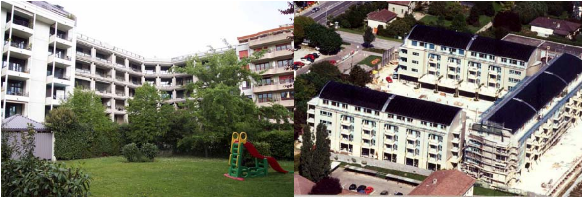
Figure 4.2 : Two HQ buildings audited within the HOPE project equipped with ground heat exchangers (photos EPFL).
