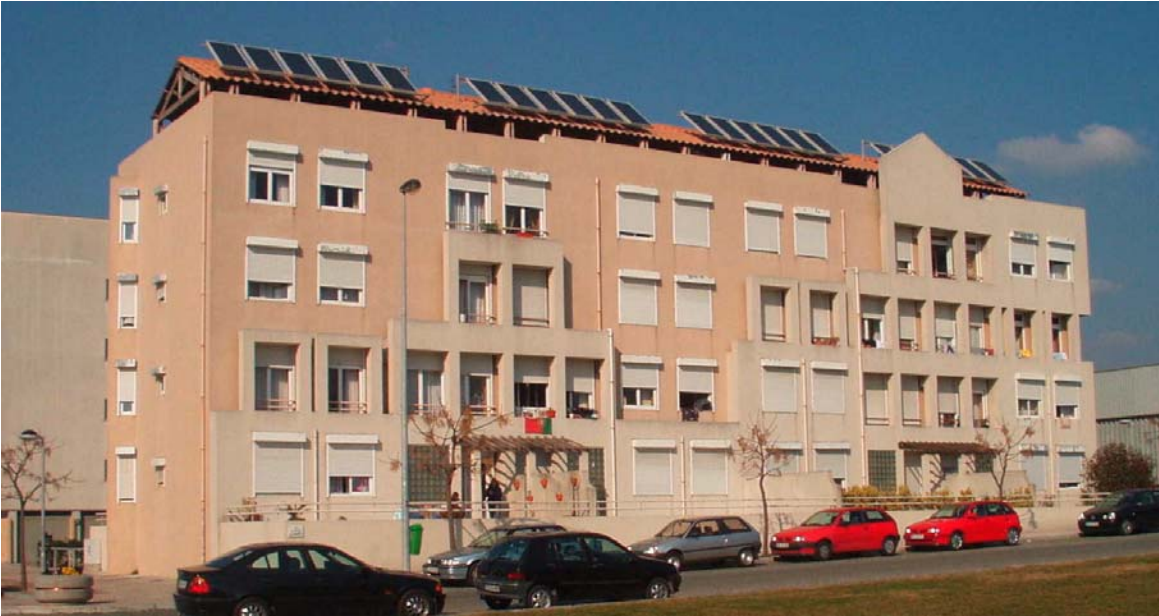
Figure 2.9: APT03 building, south facade
