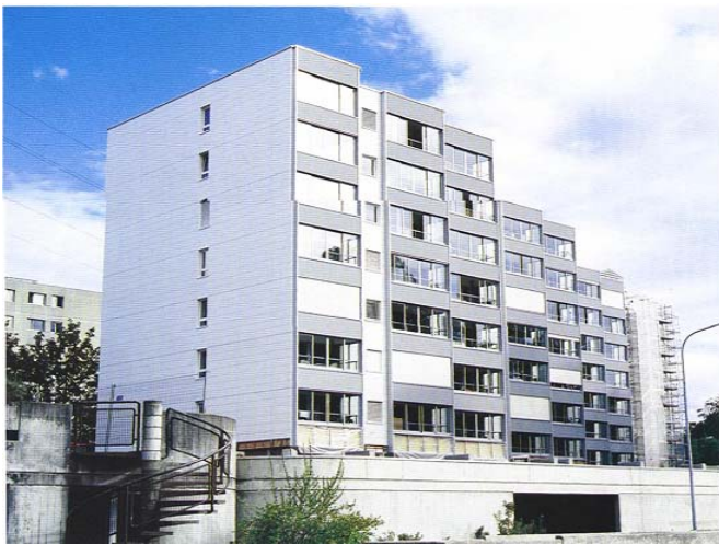
Figure 2.4: ACH03 building, seen from North-West
