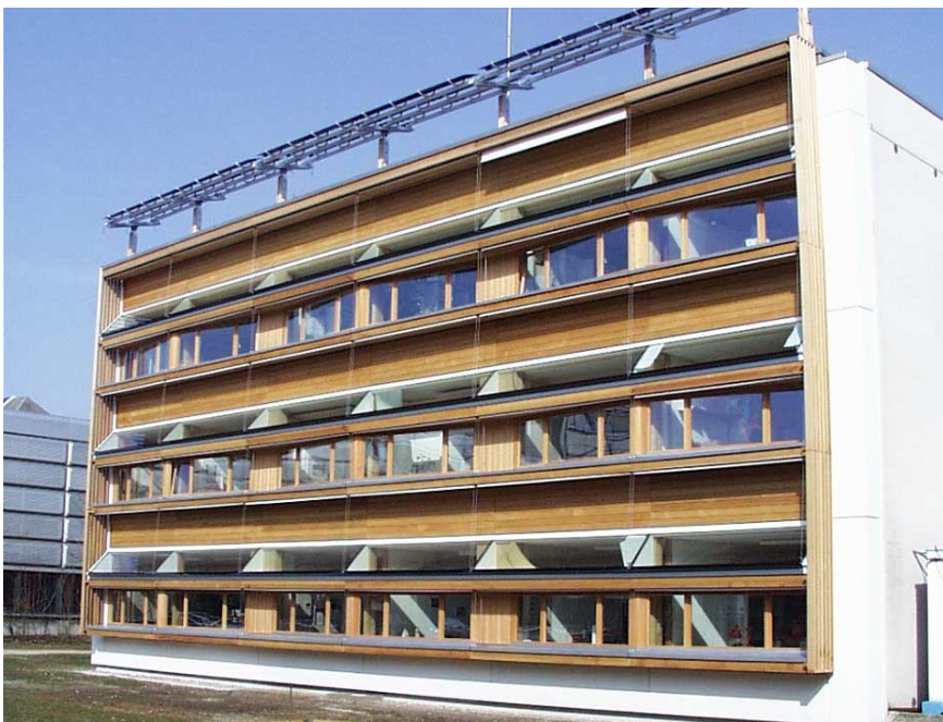
Figure 4.8 : The LESO building, in which measurements shown in Figure 4.6 were performed (Photo EPFL). This is the south façade, with large windows and special daylight devices.
