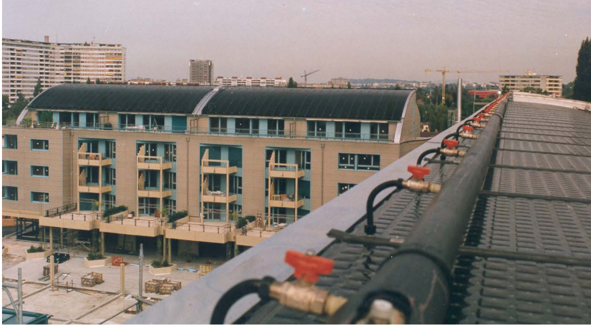
Figure 2.5: ACH06 building, with a close view on the solar roof.
